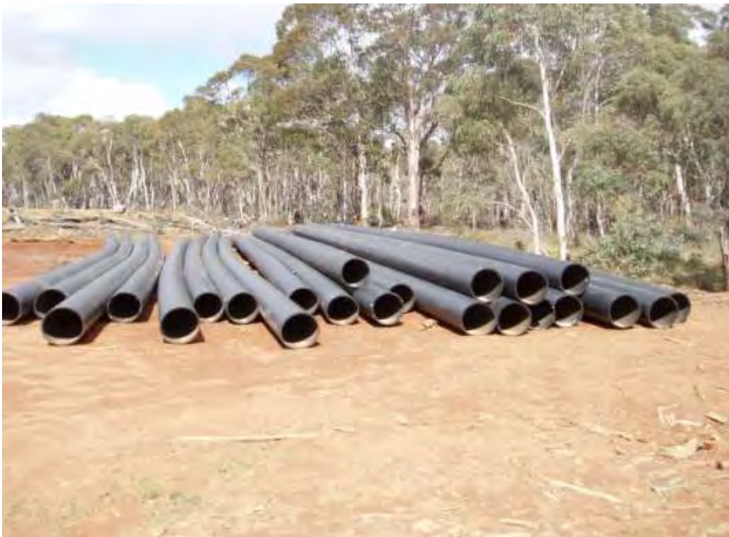
The 450mm polypipes for Springvale Colliery's pump station six on Carne Creek, which will boost mine effluent pumping rates toward 25 ML/day by 2015 (Photo: K. Muir, 2009)
