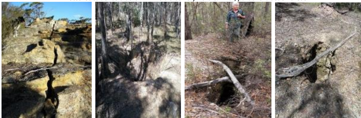
Photos: Invincible Colliery mine subsidence damage to pagodas, sinkholes, and open mineshafts
